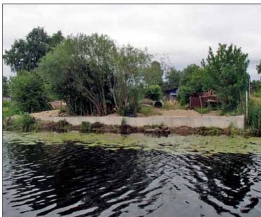
Fig. 6. Self-made protection against flood risk in the Vecdaugava River
