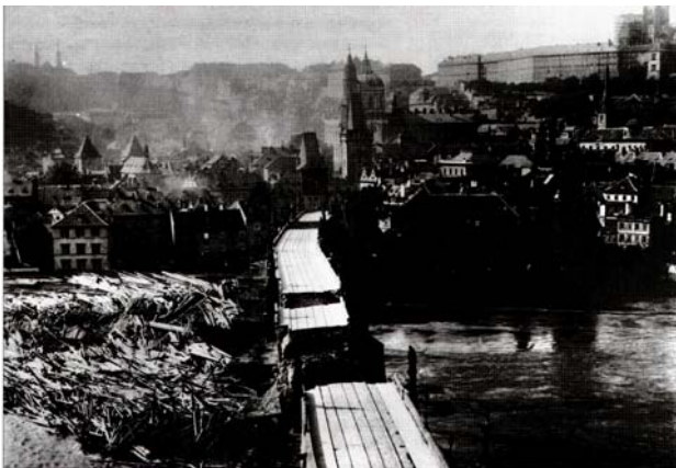
Fig 2. Collapse of 3 bridge vaults and piers of Charles Bridge during the flood of 1890
