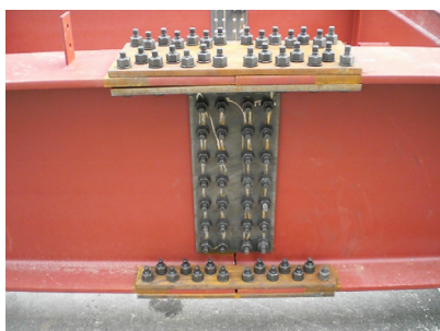
Fig. 6. An example of an existing steel connection
